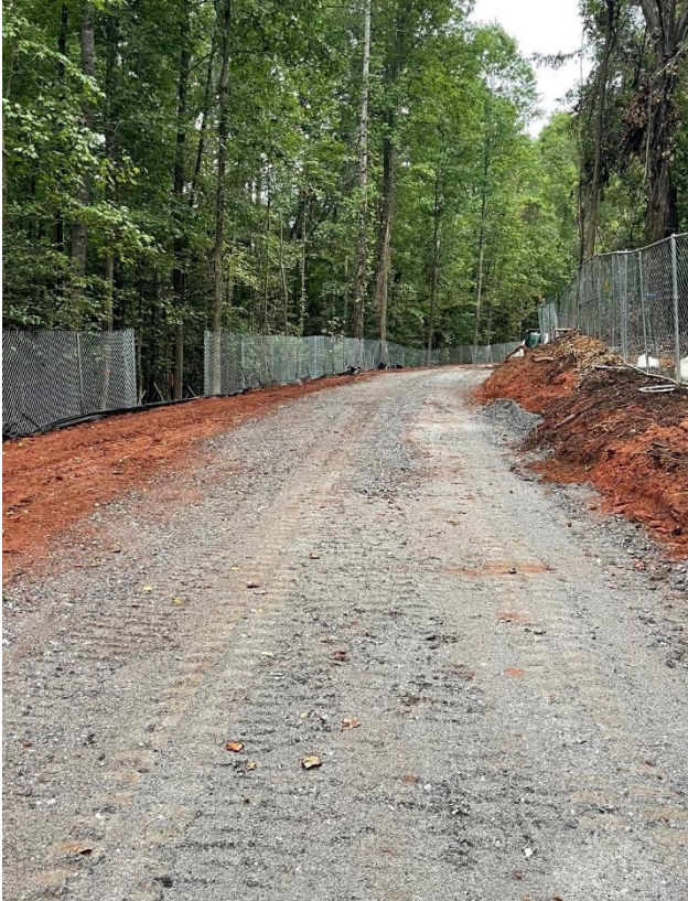
Installation of Additional Tree Protection Fencing
