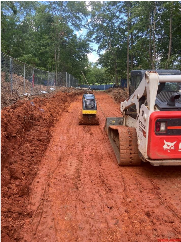
July 24 Site Grading Image
