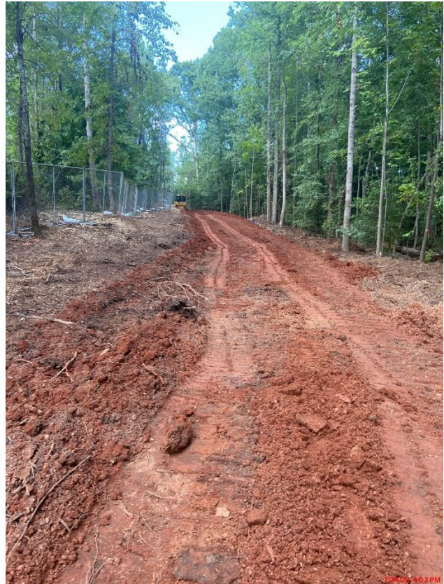
July 24 Partial Installation of Tree Protection Fencing
